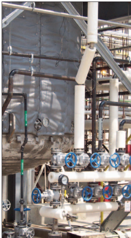
Vessel installation and piping project for Baker Petrolite.
