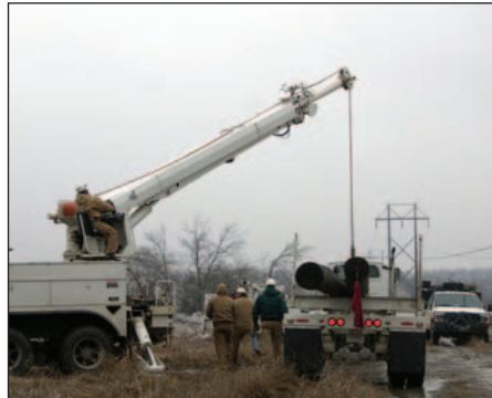
GRDA linemen unload new transmission poles, to rebuild structures near Keetonville.
