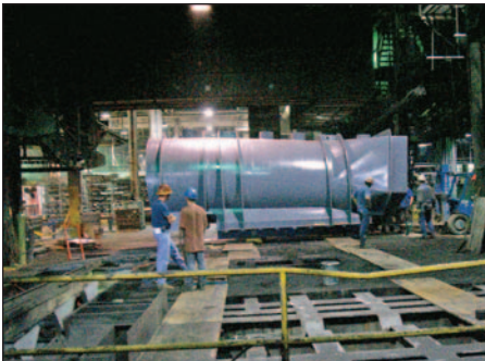
This new “Barrel Horse” was added to boost the quality of the firm’s green sand mold process.
