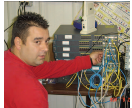
Field Engineer Chris Leatherwood configures the wireless network for Pryor. Cisco switches are used to connect the DTS network into the city's high-speed fiber optic cable.
