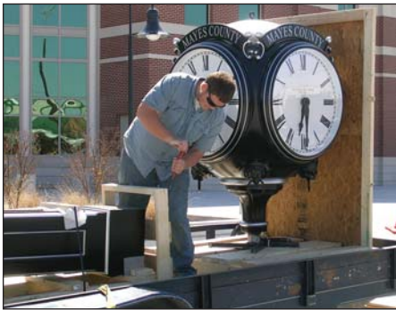
The components for the clock arrived safely on a flatbed truck.
