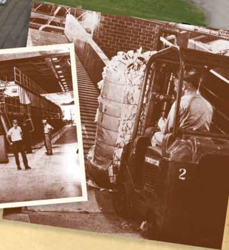
"Raw materials are carefully proportioned as they are placed on moving conveyors which feed three big disintegrating units" reads the caption to the photograph from the "Paper's New Pioneer" article about the new plant in National Gypsum News.
