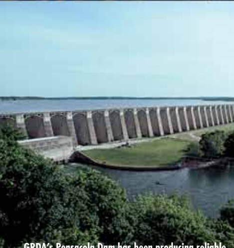
GRDA's Pensacola Dam has been producing reliable, renewable electricity since it began operations in 1940.
