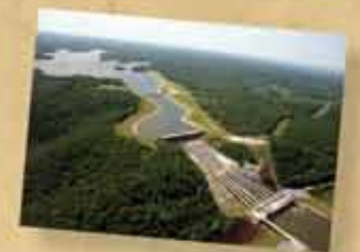
The GRDA Salina Pumped Storage Project, considered "experimental" during construction in the late 1960's, has a generation capability of 260 megawatts.
