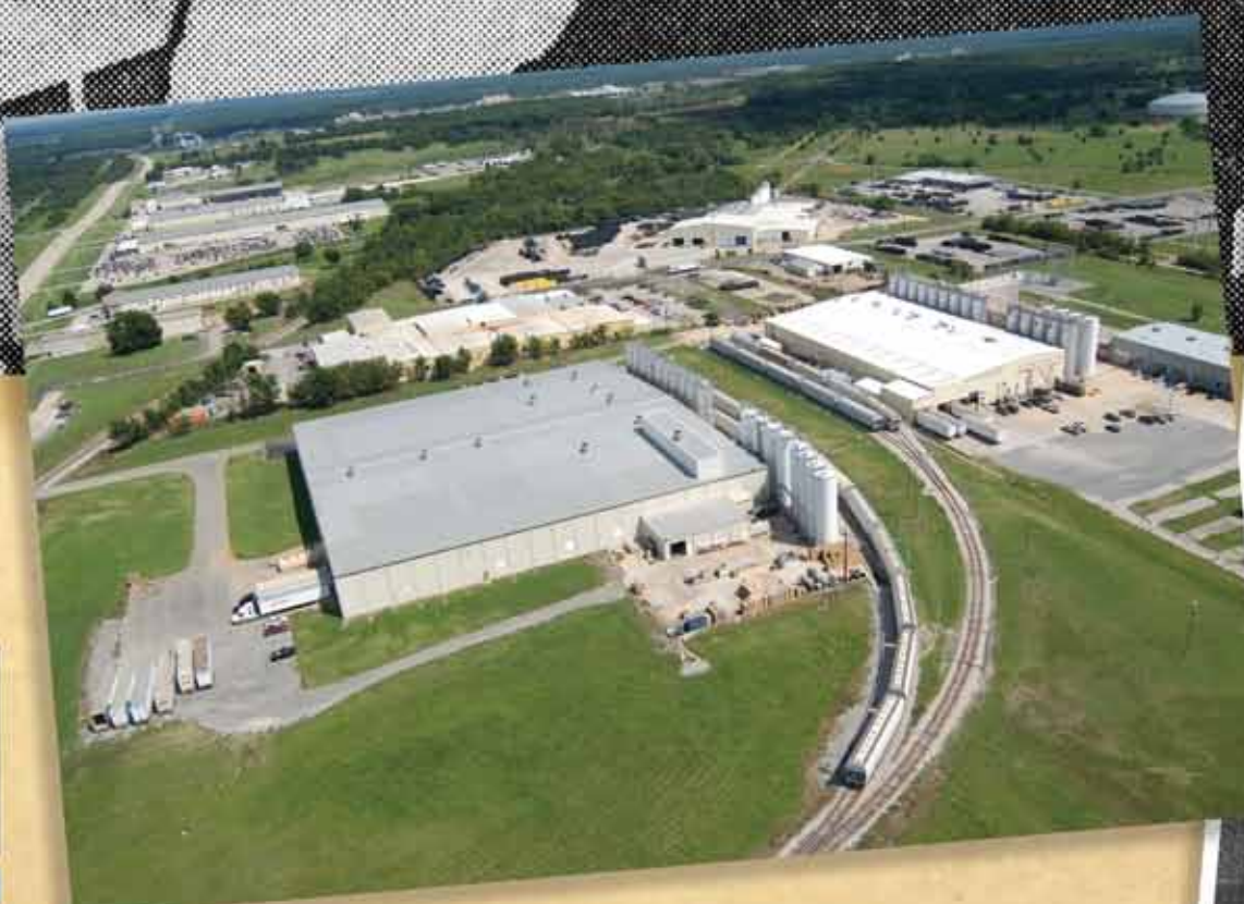
Founded in 1961, MidAmerica is a 9,000-acre manufacturing, processing, and distribution center located in Pryor Creek, Oklahoma. Regarded as the largest industrial park in the state, MidAmerica has a 365-acre airport with a 5,000-foot runway, and its own water and wastewater treatment plants. More than 80 firms are located within the park including over a dozen Global and Fortune 500 companies.
